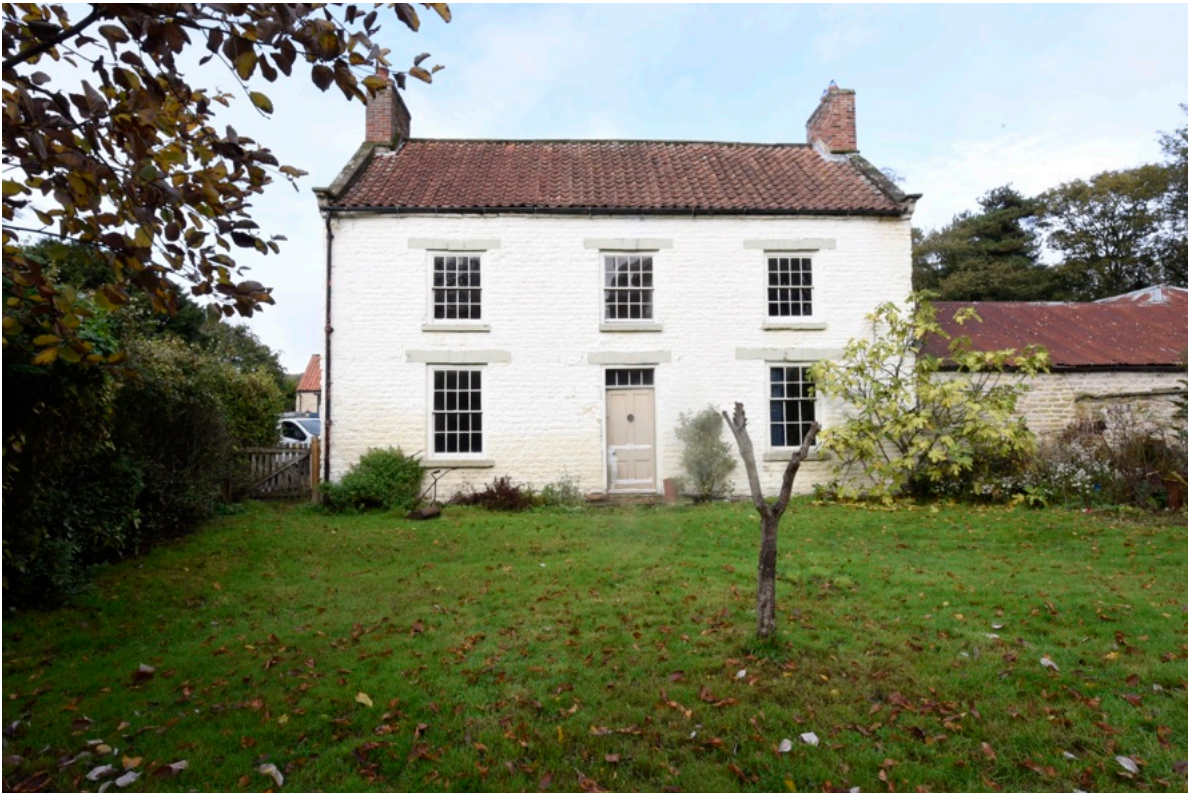
Figure 3, External Picture of Hall Farmhouse from the south.
